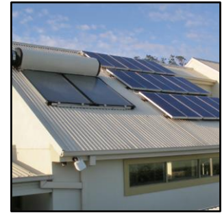
Renewable energy & storage;
