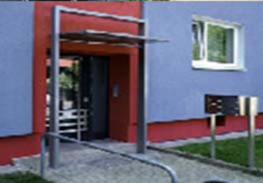
Views of new balconies and entry
