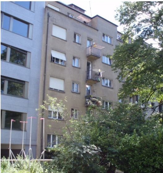
Before: courtyard facade
