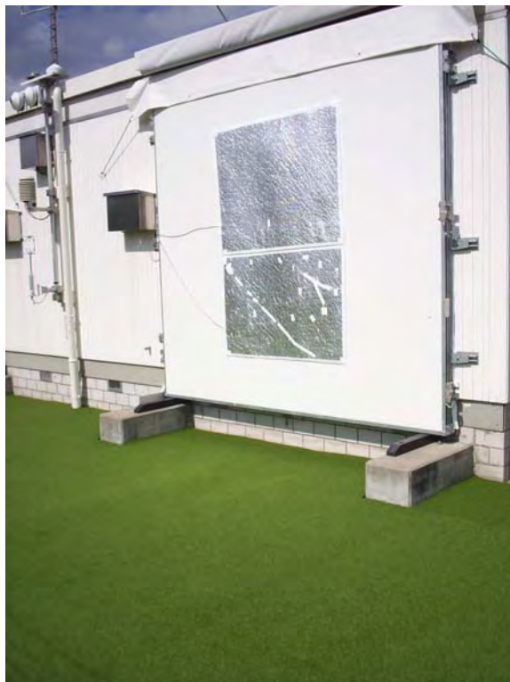
Figure 2.1. Photograph of the test cell during the preconditioning phase.
