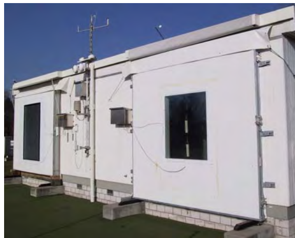
Figure 6.1. A photograph of the test cell.
