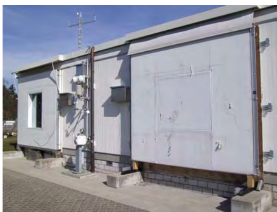
Figure 4.1b. Outdoor test facility with removable façade element.
