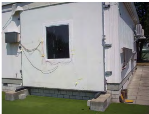
Figure 11.1. A photograph of the test cell.
