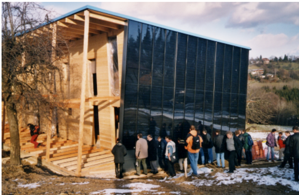
Figure 12: Two family house with a 55 m 2 collector area in the south façade
