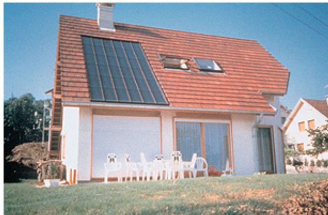
Fig. 4: French house equipped with a direct solar floor system (Source: Clipsol, France)
