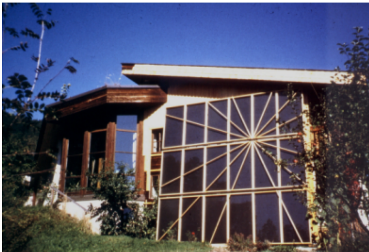
Figure 1: With the help of a façade-integrated collector it is possible to bring the sun into the façade by means of both energy and design. Source: Sonnenkraft.
