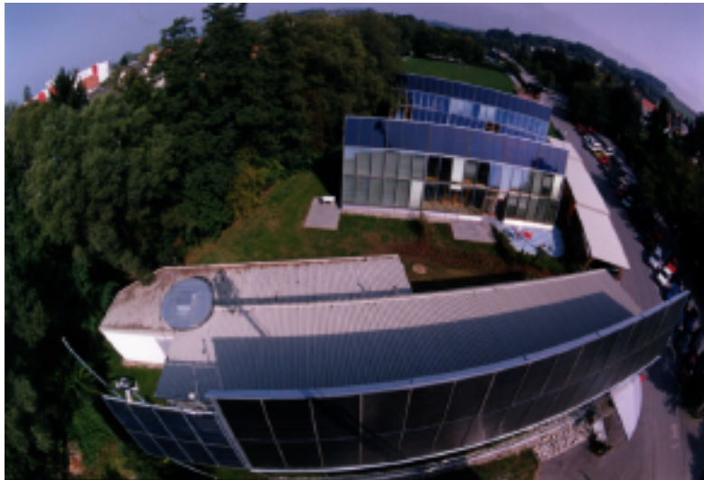
Fig.10. 60% of the space heating demand of this terraced houses are covered by solar energy (Source: AEE INTEC, Austria)
