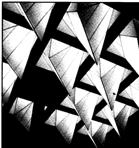
A roof system designed for daylight penetration at the Trapholt Museum in Denmark. (Lighting consultant: Sophus Frandsen)
