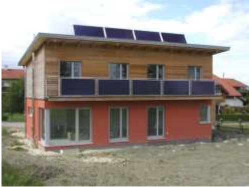
Figure 3.3.2: Single-family house in Upper Austria with two solar thermal collector arrays (on the roof and integrated in the balcony), source: AEE INTEC, Austria.
