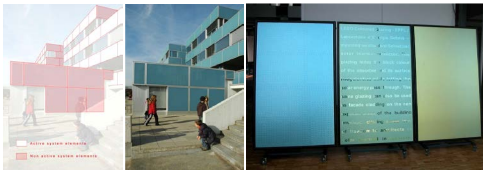
Fig. 3.1-20 left and center: Same glazing in front of active and non-active parts of a façade.
