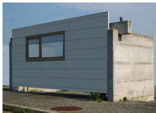
Fig. 4.6-2. Demonstration stand at Demosite-EPFL.
