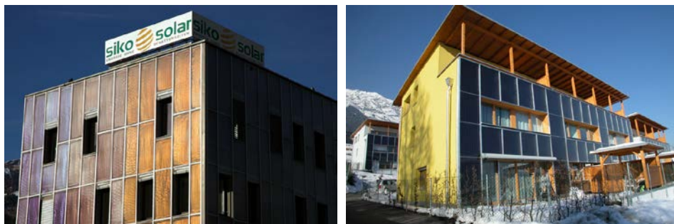
Figs 3.1-7 and 3.1-8: SIKO INTEGRAL façade collectors systems in Austria (credits: www.solar.at ).
