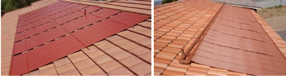
Fig. 3.2-7: Absorbers using non-selective colour material to match terracotta tiles roofing.
