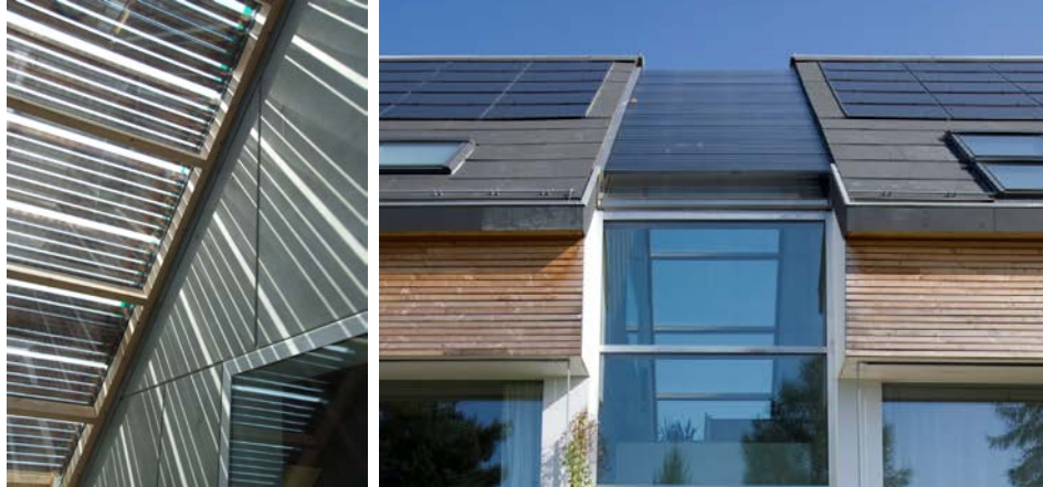
Fig.3.3-3 Evacuated tubes collectors used as glazed roof sun shading (left: inside view, right: outside view), Dübendorf residential building, Beat Kaempfen 2008.
