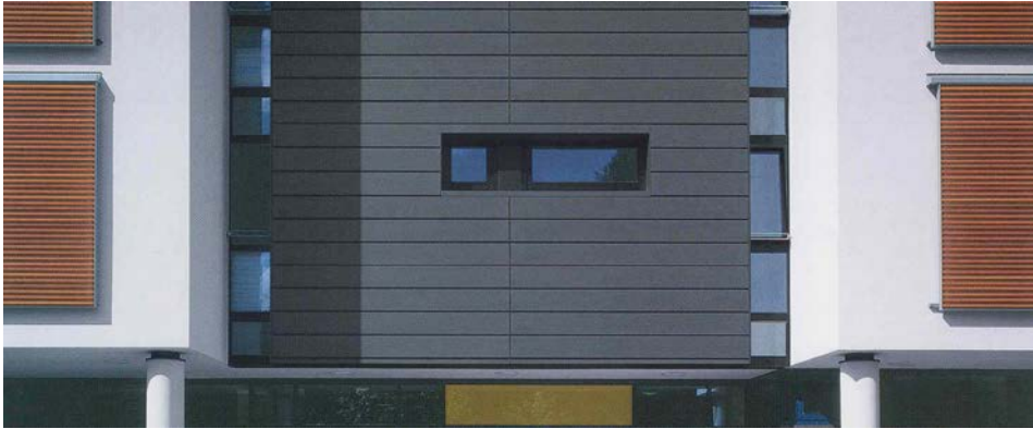
Fig. 4.5-1 Façade cladding using metallic plank system.
