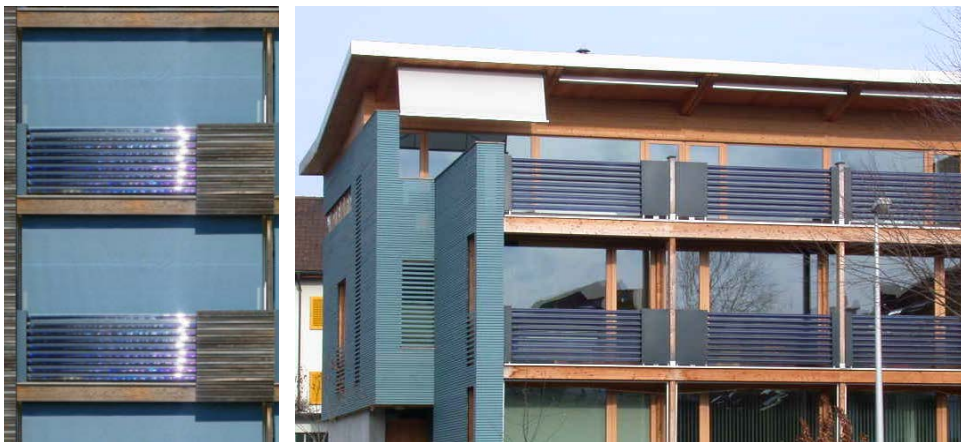
Fig. 3.3-2: Schweizer Energie vacuum tube collectors used as balcony eaves ( www.schweizer-energie.ch ), architect Beat Kaempfen, Zurich.
