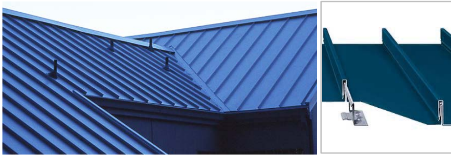
Fig 3.2- 5: Example of possible jointing solution for unglazed flat plate collectors: standing seam technique (right: standing seam technical detail).
