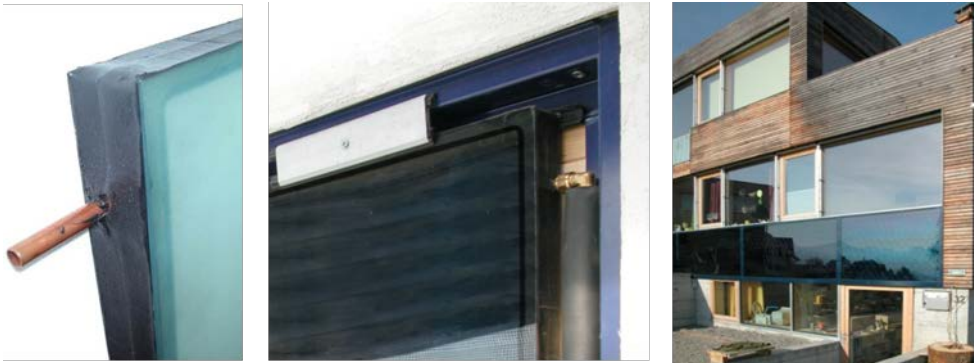
Fig. 3.1-11: Thin collectors based on triple glazing technology (H+S Solar) (see chapter 5).
