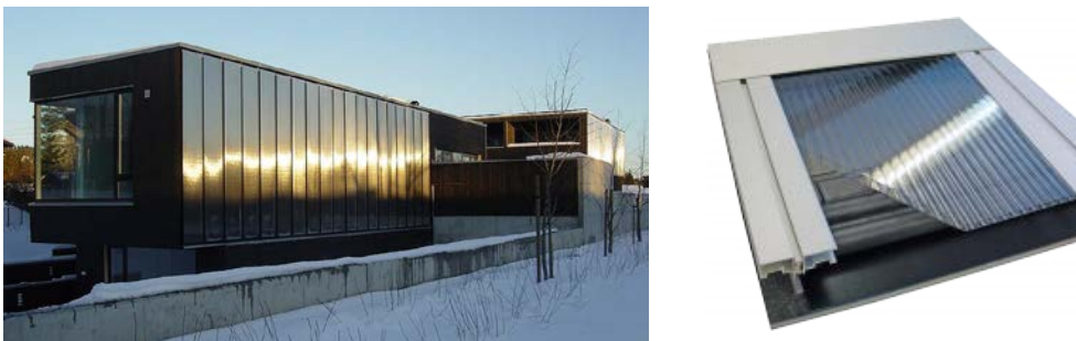
Fig. 3.1-13 Aventa polymeric collectors, facade mounted and product detail (credits: arch. Dahle/Dahle/Breitenstein AS, www.aventa.no ) (see product details in chapter 5).
