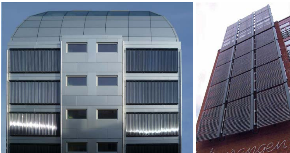
Fig. 3.3-7 left: Evacuated Tubes collectors in front of metal cladding (Hotel Swissnights Lausanne).
