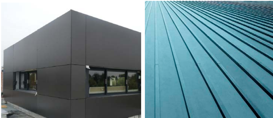
Fig. 3.2-4 left: Negative jointing between cassettes in a metallic façade cladding (Ducry SA).
