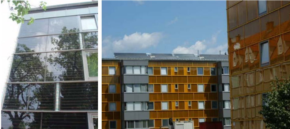
Figs. 3.1-4 and 3.1-5: Large scale prefabricated solar renovations in Austria (source : AEE-INTEC/Gap Solutions) [ http://www.estif.org/ ].
