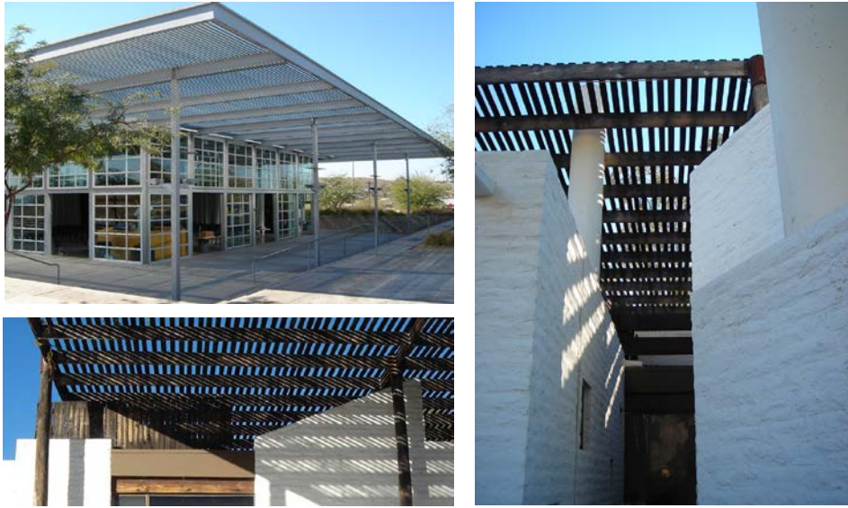
Fig. 3.3-6 a-b-c: Examples of double roofs conceived to reduce building heat (a: double tin roof in Arizona architect n.a; b and c: double roof on a private house in Arizona. Architect Judit Chafee, credits Marja Lundgren).
