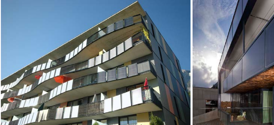
Fig. 3.1-9: SIKO INTEGRAL collectors as balcony fence ( www.solar.at ).
