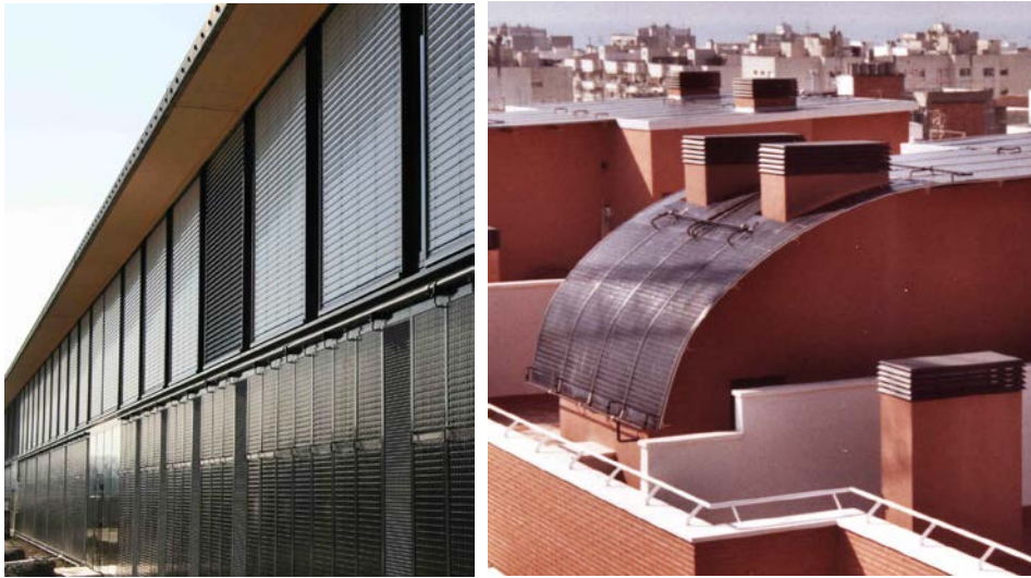
Fig. 3.2-2 left: Façade integration of unglazed flat plate collectors used as façade cladding.
