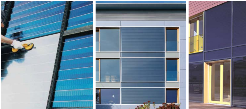
Fig. 3.1-18 a: glass fixing and jointing detail proposed by AKS Doma (VarioSol system).
