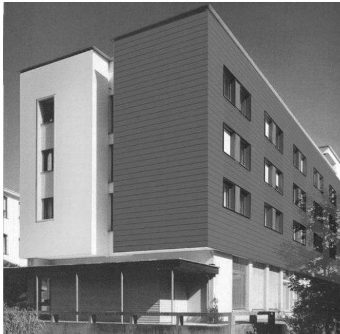
Fig. 4.7-3. New integration using the SOLABS plank.
