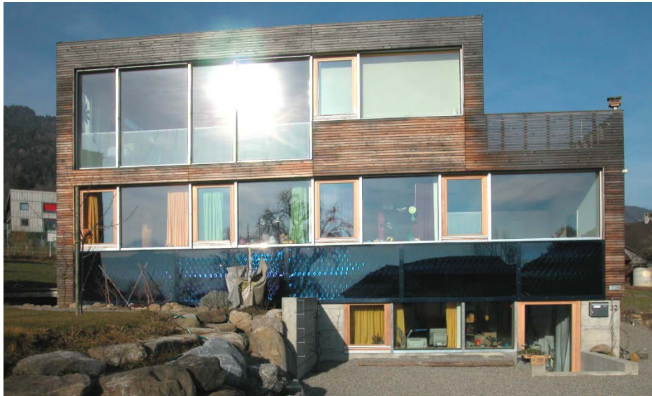
Fig. 3.1-23: Visual impact of the absorber texture under direct sunlight (Pict. H+S Hutter).
