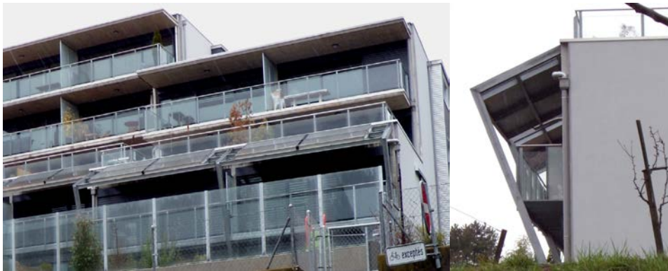
Fig. 3.1-10: Glazed flat plate collectors used as sun shading systems (credits EPFL-LESO).
