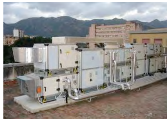
Figure 5. Sketch of the system and the installation of the air-handling unit of the solar assisted DEC-System at the University of Palermo in Italy (source: DREAM).
