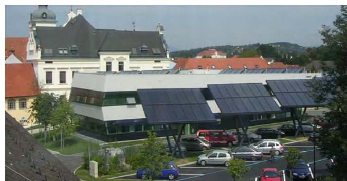
Figure 4. Solar heating and cooling installation at the Town Hall in Gleisdorf, Austria (304 m 2 flat plate collectors connected to 35 kW Yazaki chiller WFC 10 and a desiccant evaporative cooling system). (Source: AEE INTEC, Gleisdorf)
