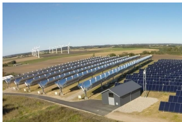
Figure 6: Combination of flat plate collectors and parabolic trough collectors in Taars, Denmark (Aalborg CSP)
