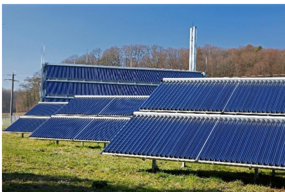
Figure 5: Ground mounted evacuated tube collectors in Büsingen, Germany (Solites)
