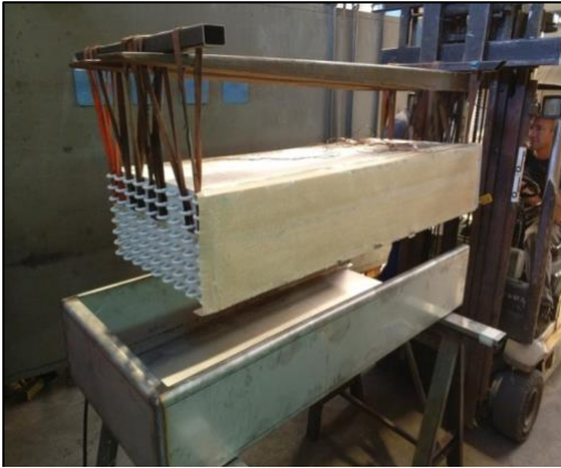
The interior heat exchanger is lifted into the prismatic containment.
