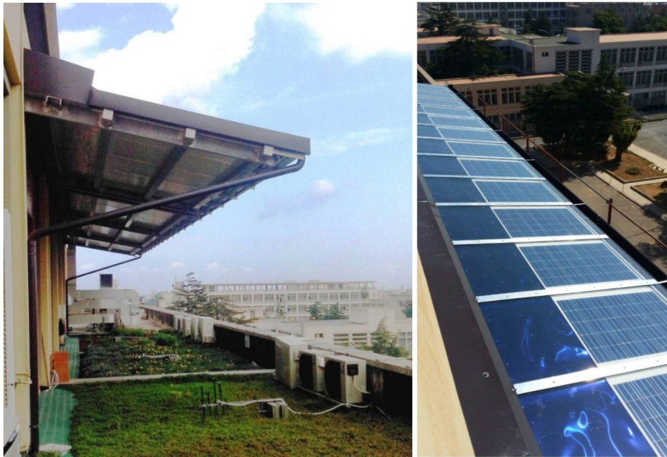
Figure 2.6.1.2: Hybrid photovoltaic/thermal (PV/T) collectors
