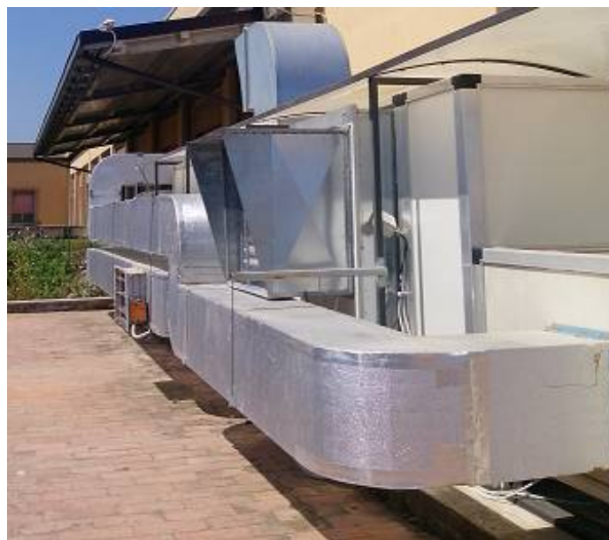
Figure 2.6.1.1: Solar assisted AHU-DEC
