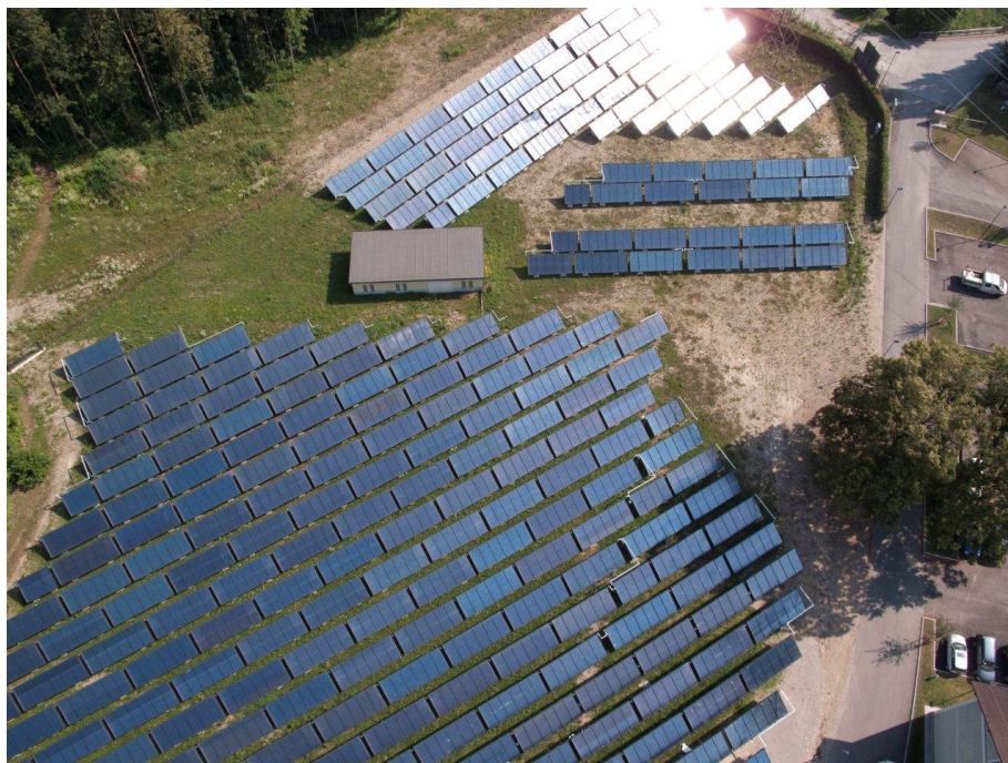
Figure 14. ST collector field at Wasserwerke Andritz in Graz (Austria)
