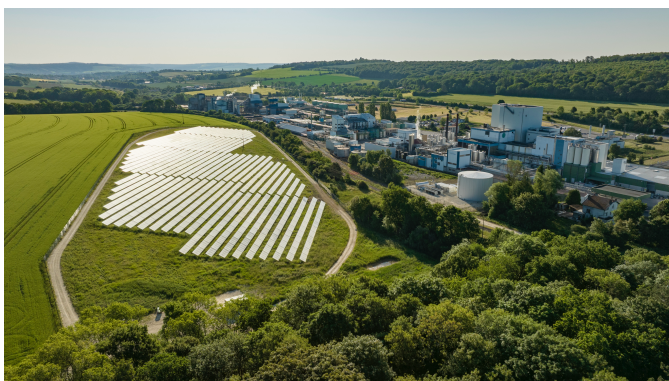
Project: NEWHEAT. Photo credit: IMAGESinAIR
