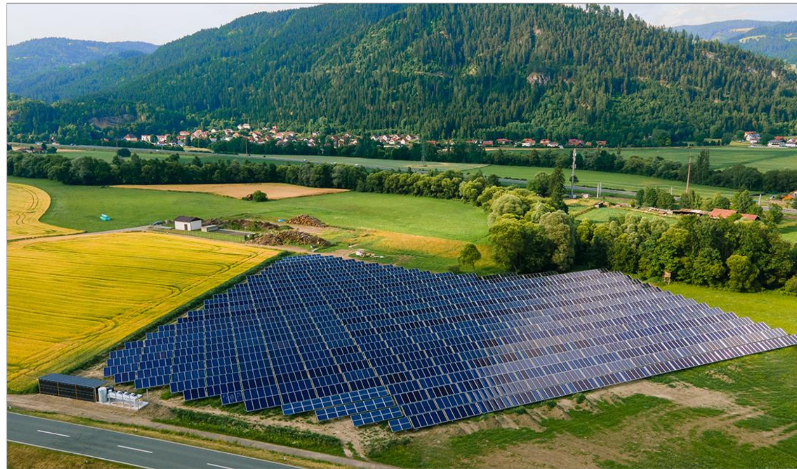
Friesach, Source: Solar Engineering Guggenberger
